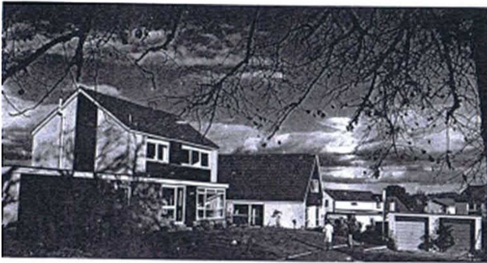
Figure 40.4 Housing at Park Way in Kildrum.
